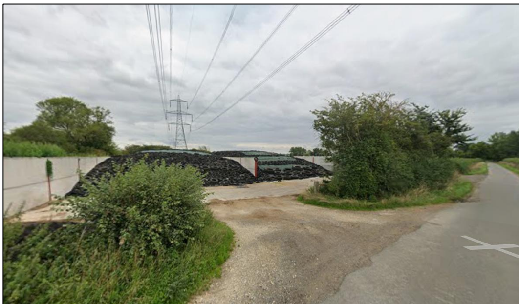
Figure 6: Existing Silage Clamp Access
